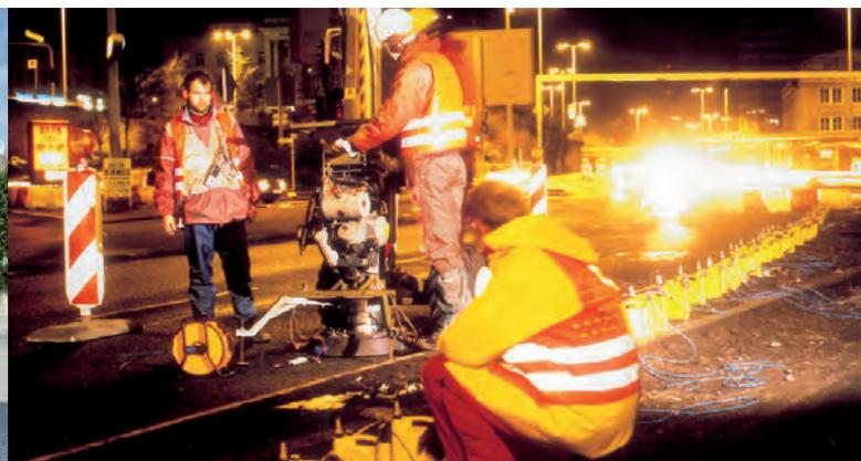
Investigation and localisation of road setup and components via ground penetrating radar
